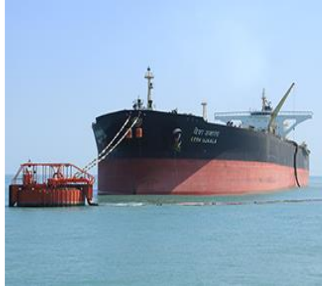
Single Point Mooring
